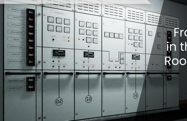
From the main switchboard in the vessel's Engine Control Room, the user has to restore power by starting and synchronising generators manually.
